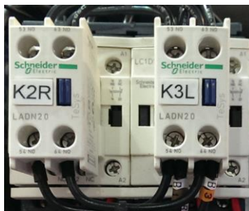
Reversing contactors with mechanical interlock
