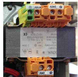
Transformer input 415V 3ph Output 24vac
