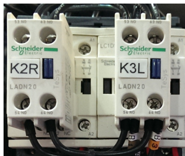
Reversing contactors with mechanical interlock
