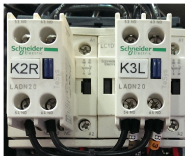
Reversing contactors with mechanical interlock
