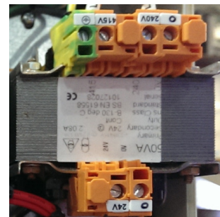
Transformer input 240V 1ph or 415V 3ph - Output 24VAC
